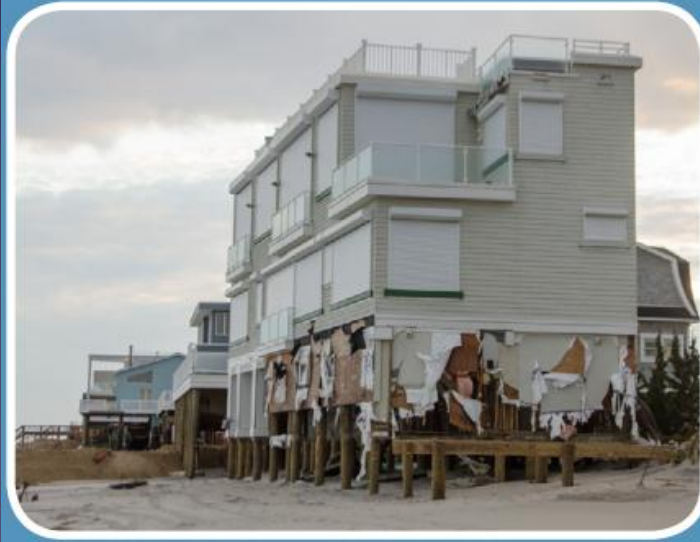
Hurricane Sandy moved sand off the beach and ocean water undermined beachfront properties.
