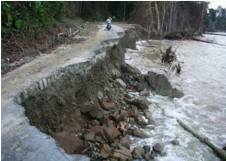
Figure 3. Channelized scour. Great Nicobar Case RS-3.
