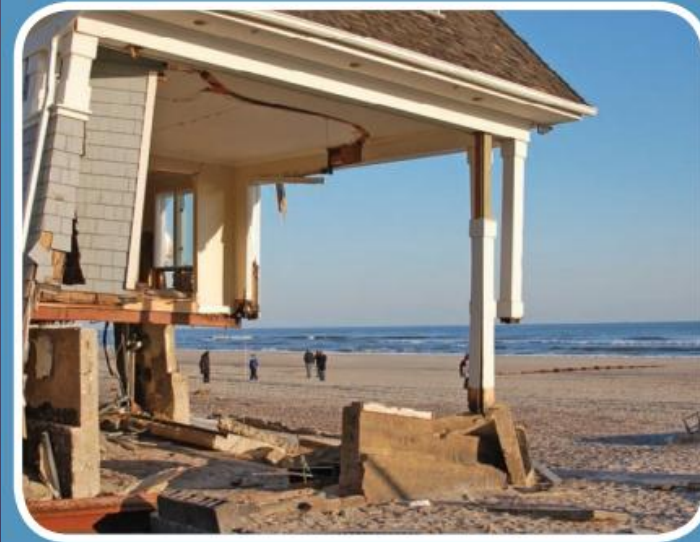
Wave, storm surge and erosion damage to oceanfront house in Belle Harbor, Rockaway, NY.
