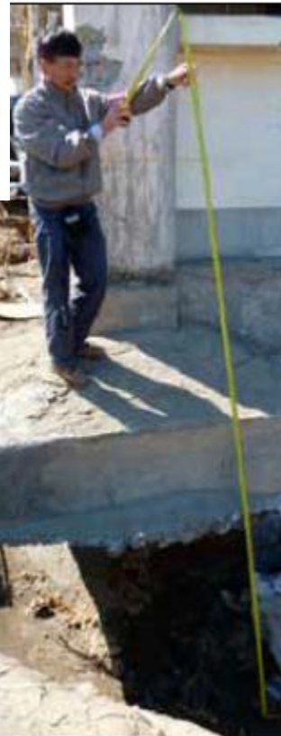
Figure 28. Gary Chock measures the depth of scour below a building corner (photo: Robertson/ASCE).
