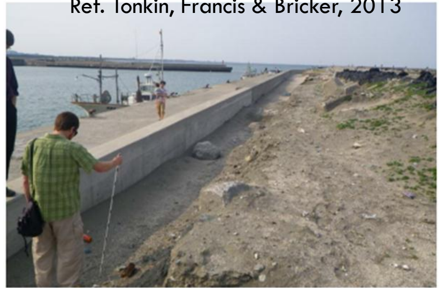
Figure 2. Overtopping scour, Taito Port, Japan. Case TO-1.
