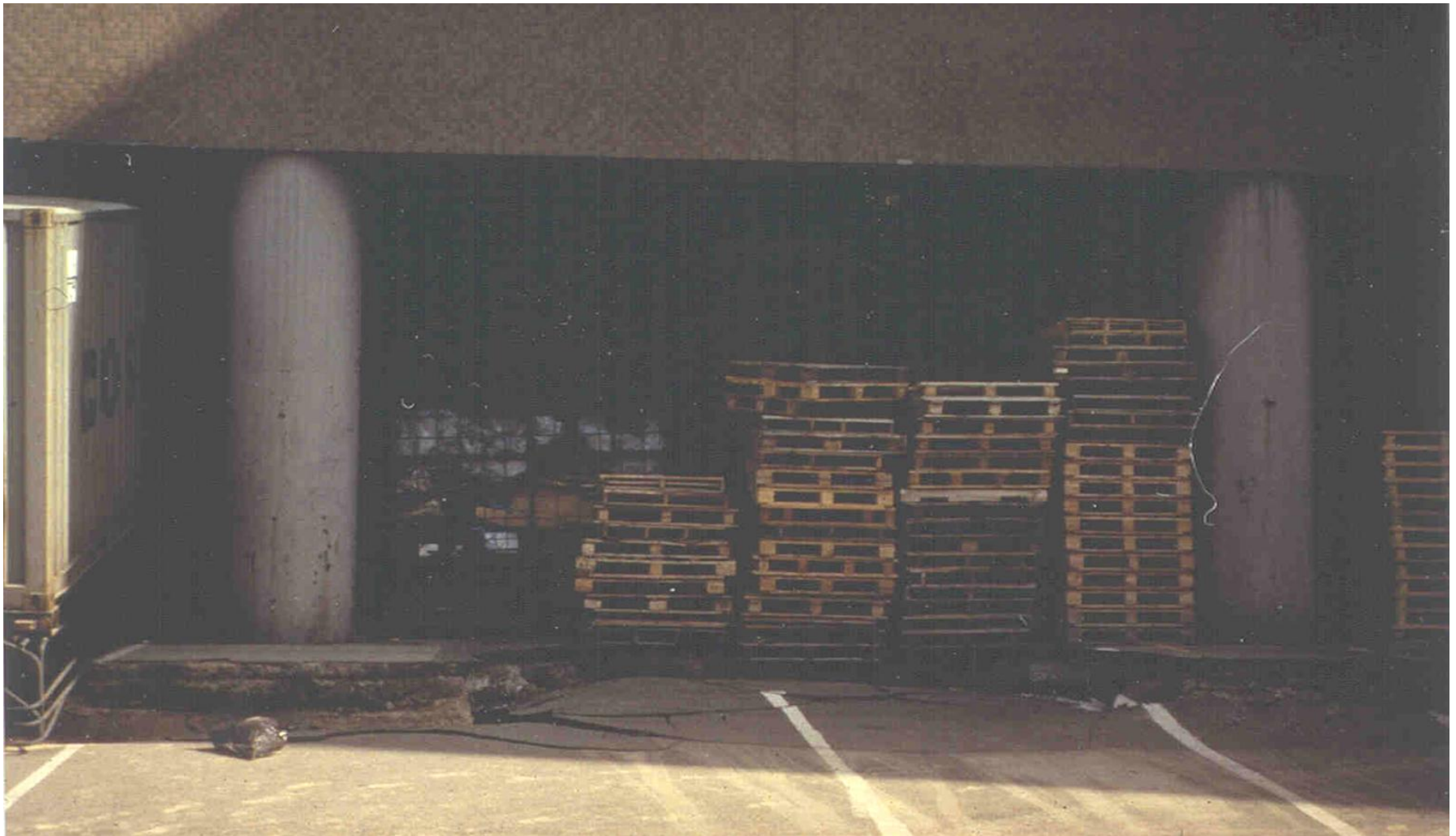
0.5 m of differential settlement between building, founded on piles, and ground caused no significant structural damage; Port Island, Kobe, Japan (Les Youd photo)
