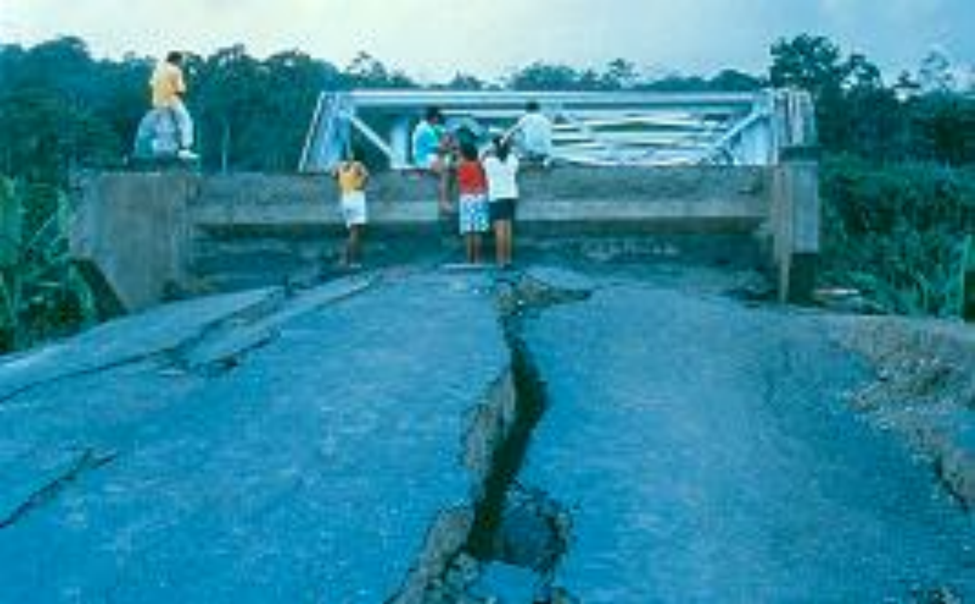
Cracked and settled highway embankment at abutment of collapsed Rio Estrella highway bridge (University of Costa Rica photo)
