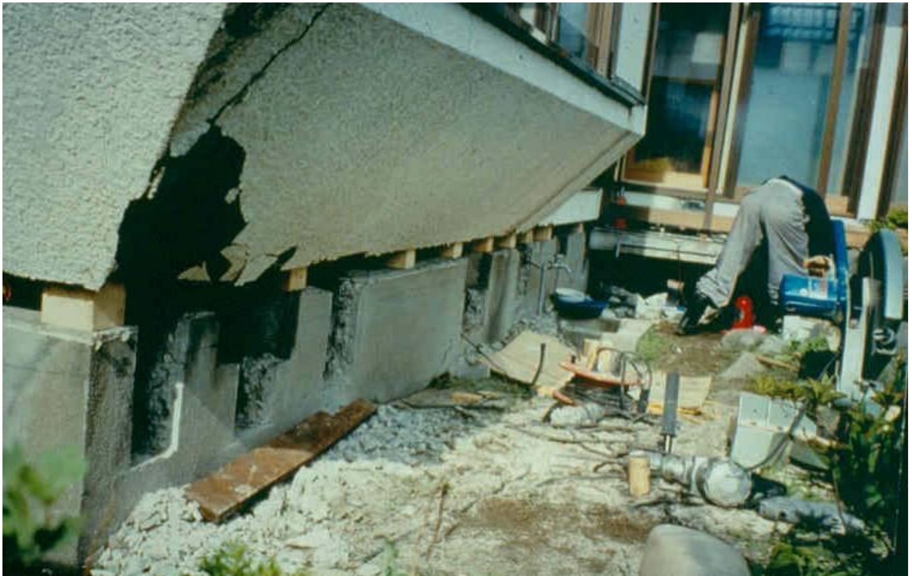
House in liquefaction and lateral spread zone that tilted, but was undamaged structurally during 1993 Hokkaido, Japan earthquake; house undergoing re-leveling (Les Youd Photo)
