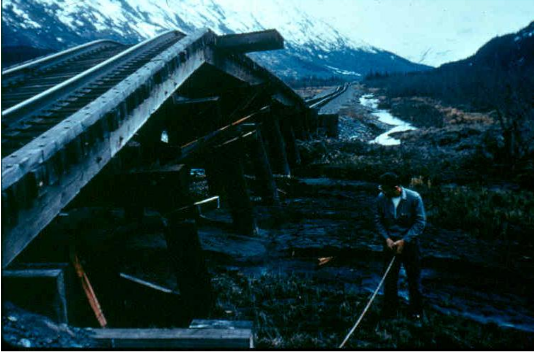
1964 Alaska earthquake: lateral spread floodplain deposits displaced abutments 1 m toward channel buckling deck upward (USGS photo)
