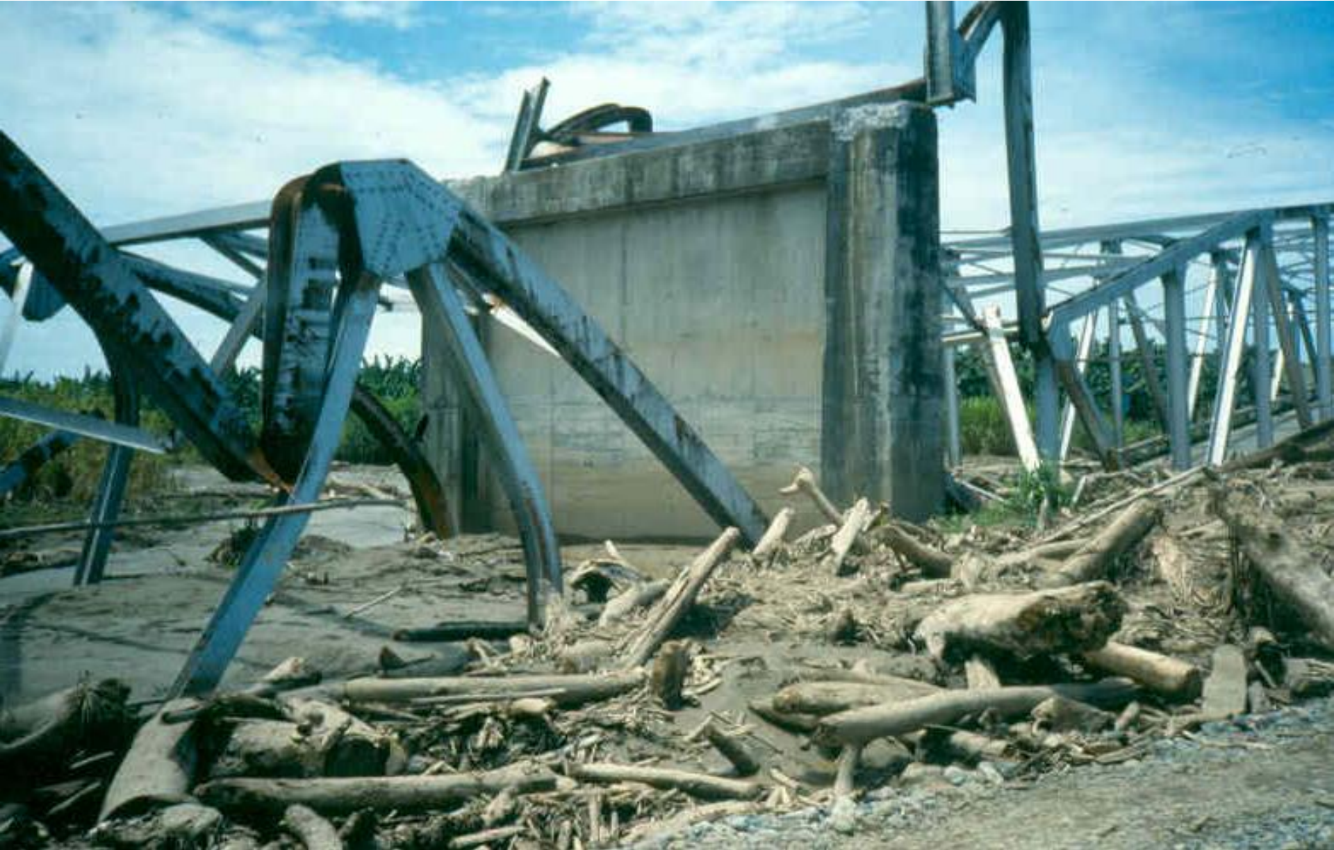
1991 Limon Costa Rica: Central pier of Rio Estrella highway bridge
