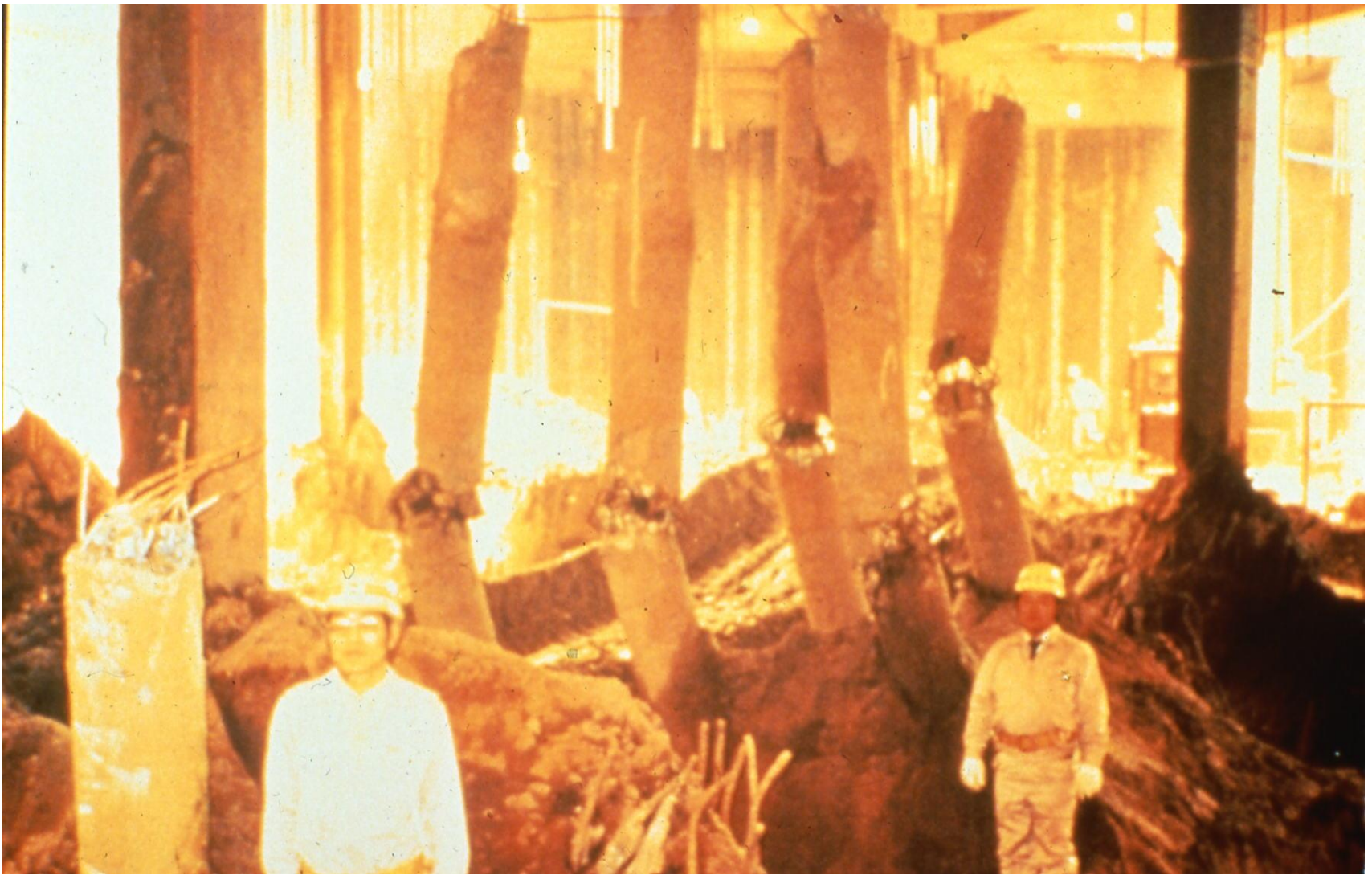
Fractured Piles Beneath N Building exposed during excavation for a new building in 1985; damage to piles caused by Lateral Spread during 1964 Niigata, Japan Earthquake (Japanese contractor photo)
