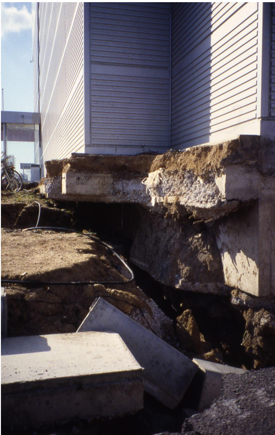
Waterfront side of Ferry Building showing pavement that settled and pulled away from building due to liquefaction and lateral spread, exposing foundation elements (Les Youd photo)
