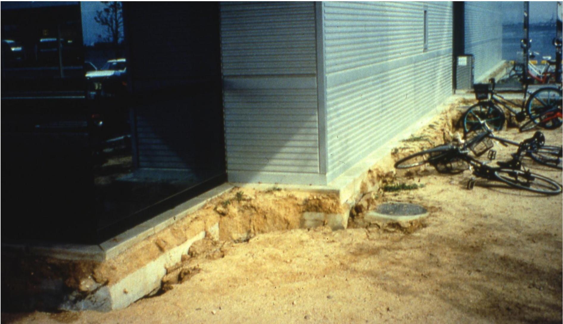
Ground settled approximately 0.5 m around Ferry Building (Les Youd photo)
