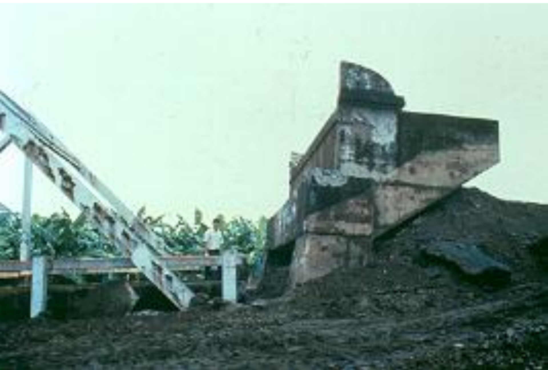
Abutment and collapsed truss of Rio Estrella highway bridge (University of Costa Rica photo)
