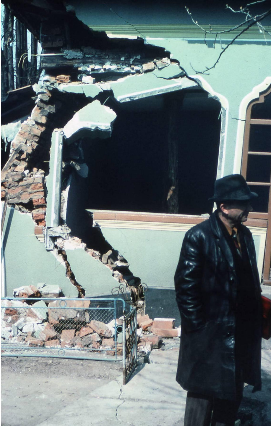
House pulled apart at the foundation level by lateral spread; 977 Varancia, Romania earthquake (Lloyd Cluff Photo)
