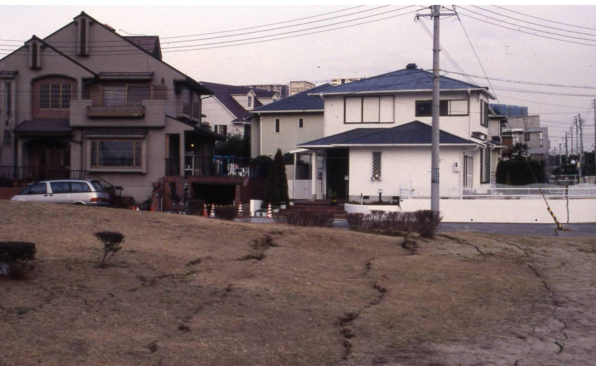
Liquefaction-generated lateral spread fissures during 1995 Kobe, Japan earthquake; the fissures pass beneath houses but caused no damage (Photo by Nick Sitar)
