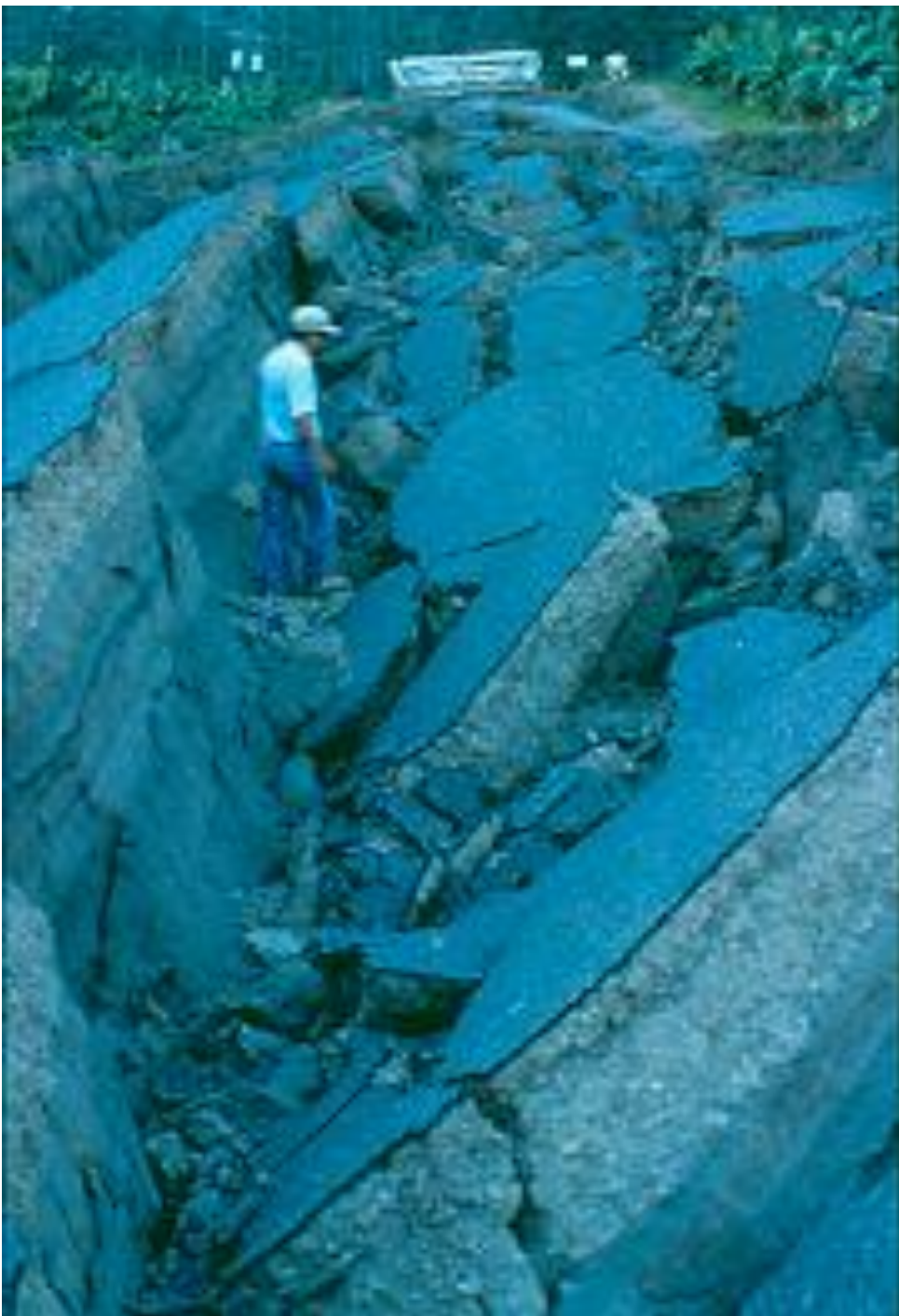
Shattered and spread embankment approach to collapsed Rio Estrella highway bridge (Univ. of Costa Rica photo)
