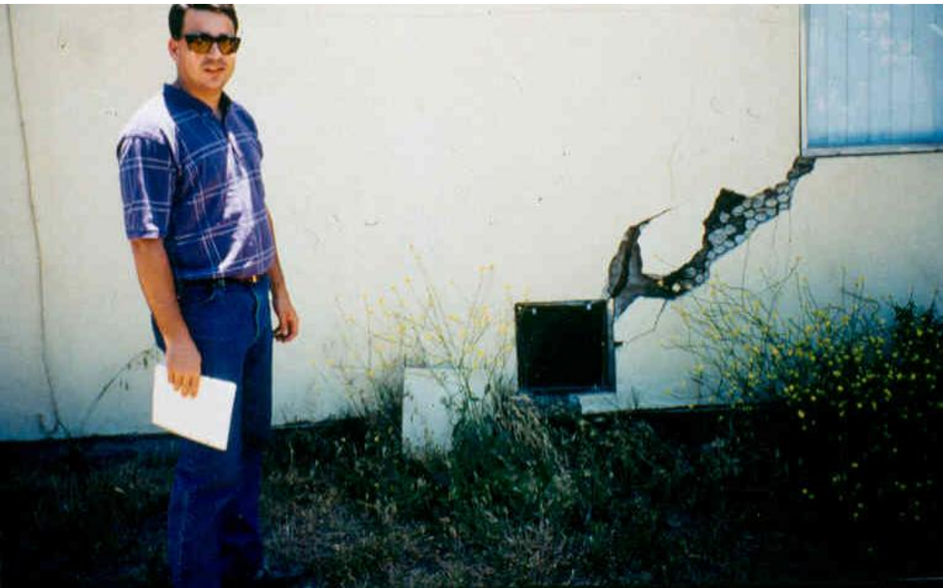
House in Sylmar, California that pulled apart by lateral spread during 1995 Northridge earthquake (Les Youd Photo)
