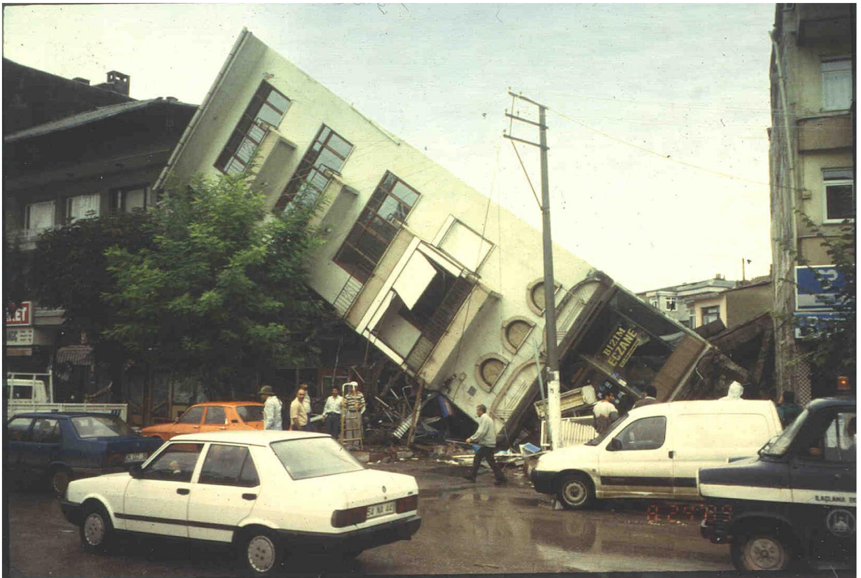
Tipped building in Adapazari, Turkey caused by liquefaction-induced loss of bearing strength during 1999 Koaceli, Turkey earthquake (Les Youd photo)
