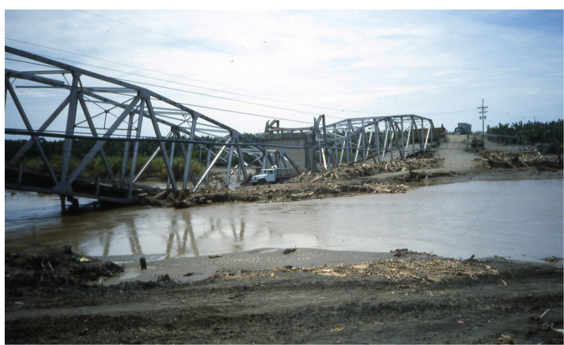
Collapsed highway bridge over Rio Estrella, 1991 Limon Costa Rica earthquake (Les Youd photo)
