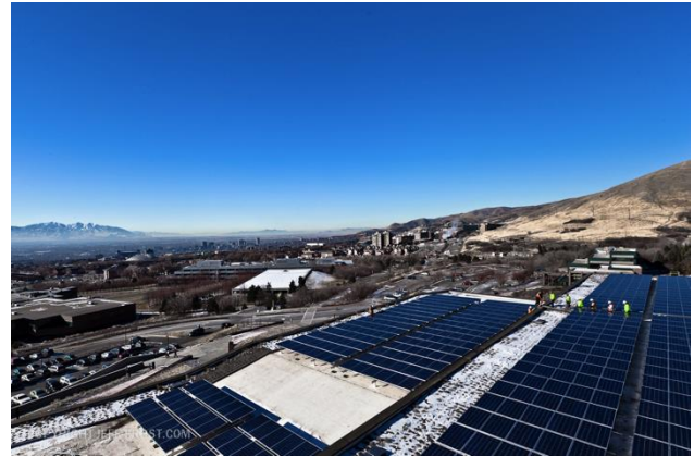
A 330 kilowatt solar installation at the Natural History Museum of Utah. Utah's solar capacity has grown rapidly in recent years. Retrofitting existing solar installations with battery storage can provide resilient backup power in the event of a grid outage. 1
